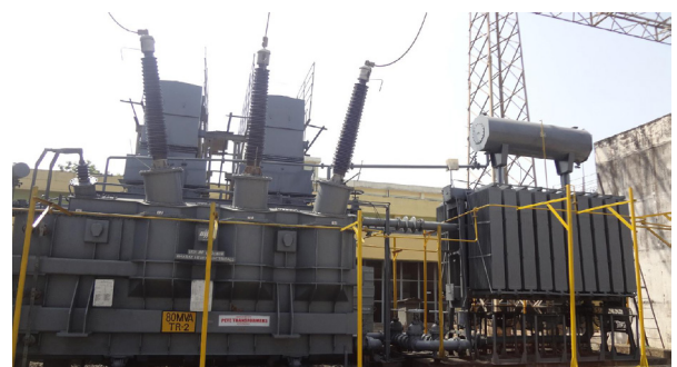
On-site servicing of 220kV Class Transformer
