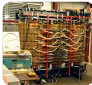
TEMPERATURE RISE TEST
