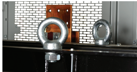
Lifting eyes for core & coil assembly
